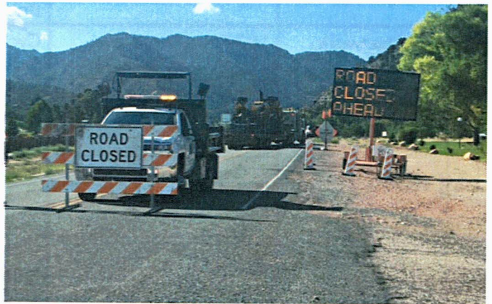
Construction in Parowan Canyon (Holmes, 2017)
