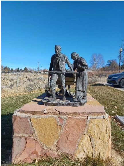
Bodil Mortensen Tribute by Stanley J. Watts. Bronze. Needs immediate attention. Façade stones are loose and loosening.
